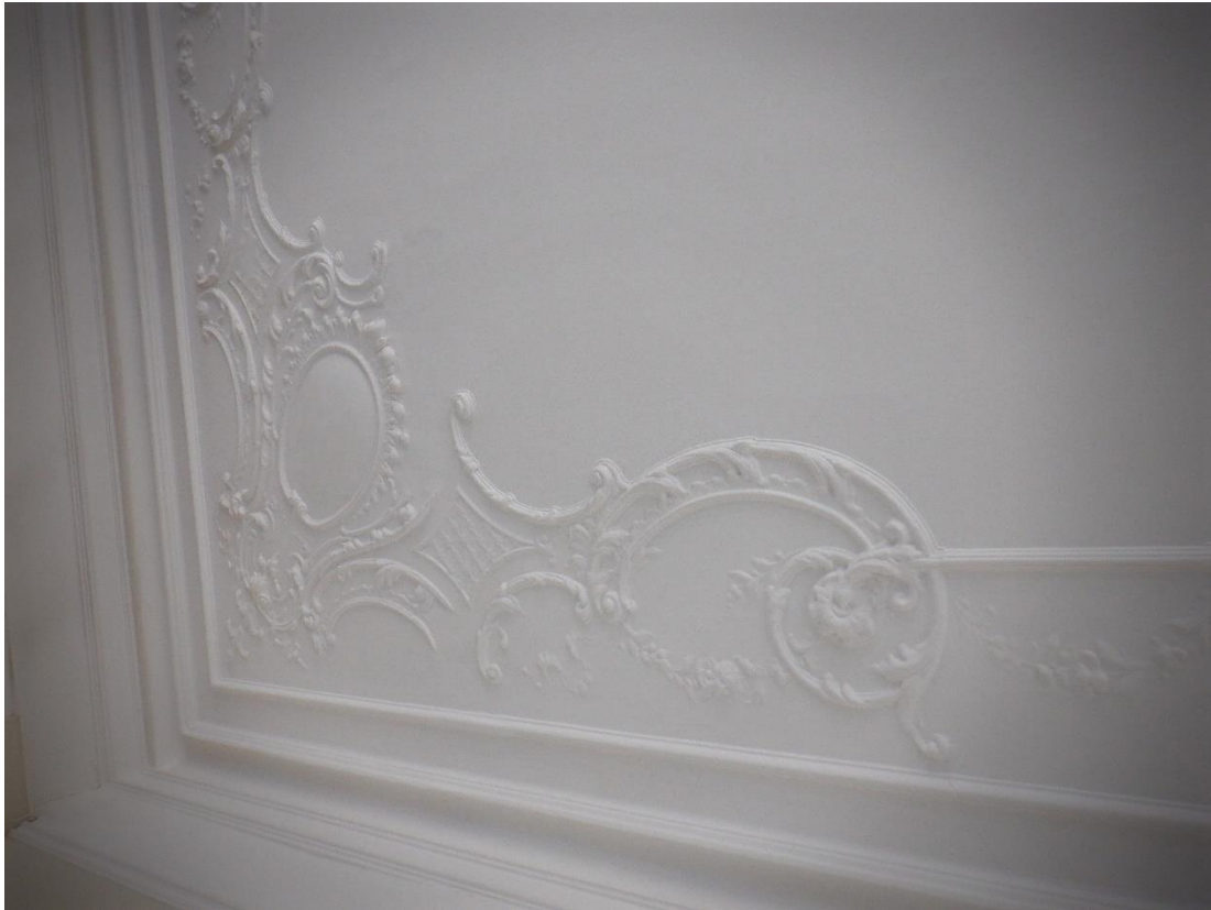
Plate 11. Detail of plaster ceiling mouldings
