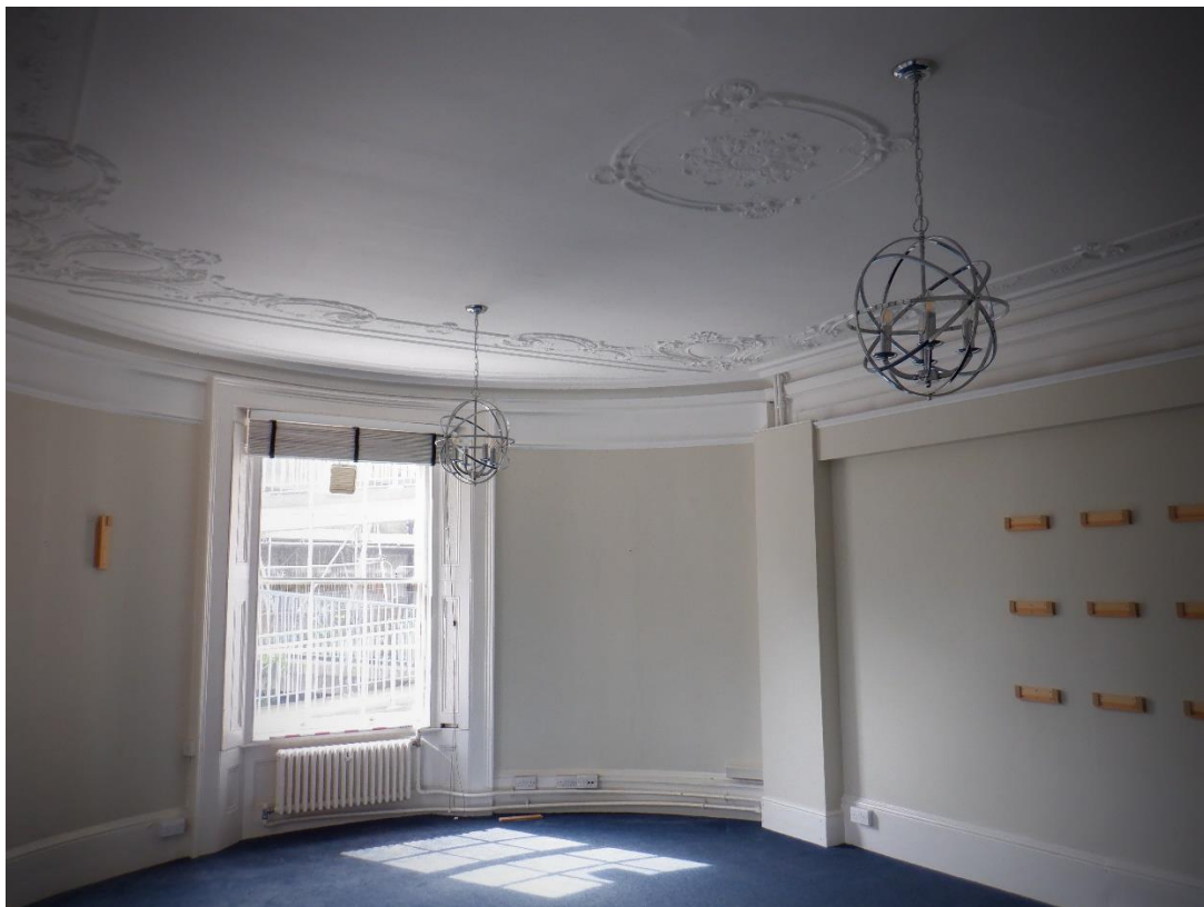
Plate 10. Plaster decoration with ceiling rose, coving, cornice and panel moulding
